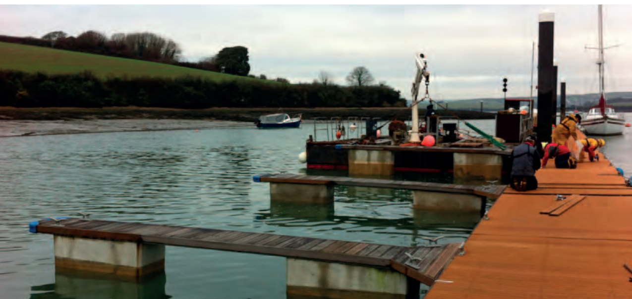
Harbour staff fitting four fingers to B Pontoon in Coad Cove. These fingers will be used for vessels up to 8m LOA
